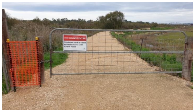
Photo: Restricted access to levee banks.
